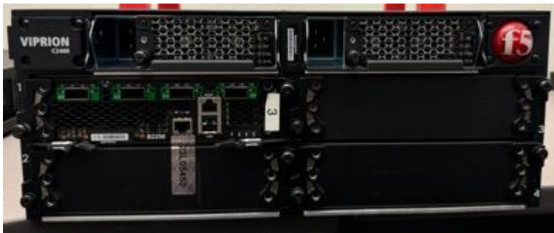
Figure 6 - B2250 blade mounted in VIPRION chassis C2400 with three blanks
